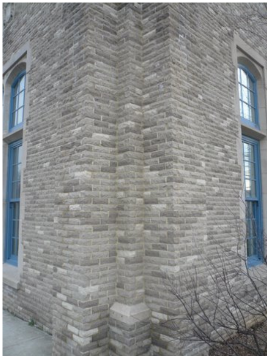
Isaac Young Middle School, New Rochelle, NY Gray Rockface Brick Blend 34% pre-consumer waste
