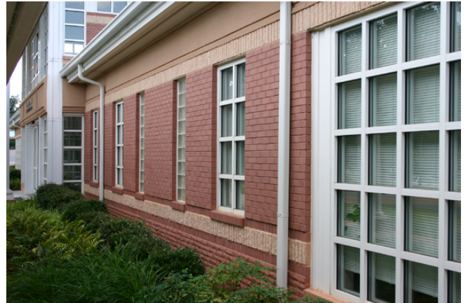
Kings Mountain Senior Center in Kings Mountain, NC Baystone modular size brick 55.1% pre-consumer waste Coral modular size brick 65.8% pre-consumer waste
